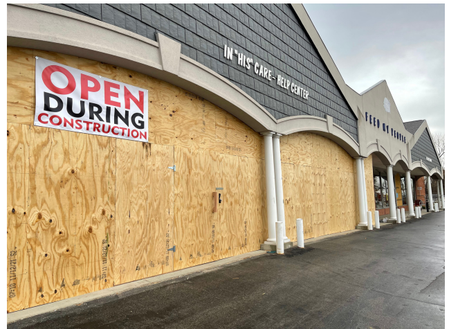
Current FMP construction work.
